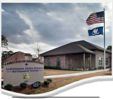
Louisiana State Police Retirement System Building located at 9224 Jefferson Hwy, Baton Rouge, LA 70809
